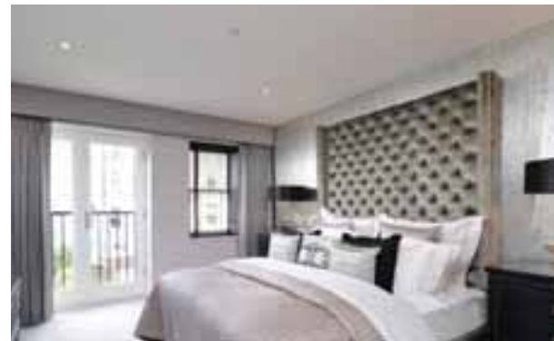
Room with concealed sprinkler head (image courtesy of St James).
